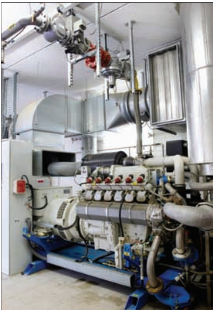
Figure 1 Improving reliability of rotating equipment in biodiesel facilities with PCS systems has substantial benefits, even for small plants
